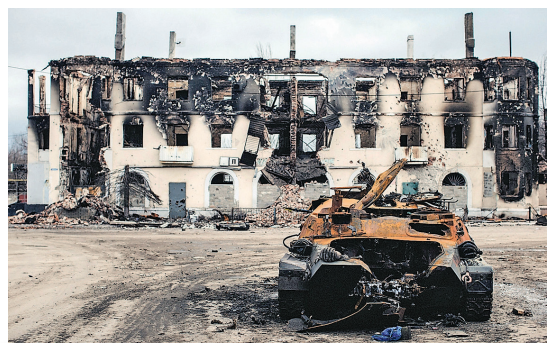
The remains of a tank outside the remains of an apartment building in Vuhlehirsk, February 2015. Photo by Max Avdeev for BuzzFeed News Source: https://www.buzzfeed.com/gabrielsanchez/pictures-from-the-front-lines-of-ukraine
